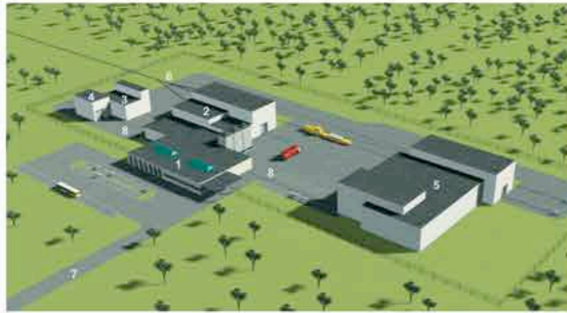
Components of a geological repository for spent fuel (SF), high-level waste (HLW) and long-lived intermediate-level waste (ILW), presented in model form.
